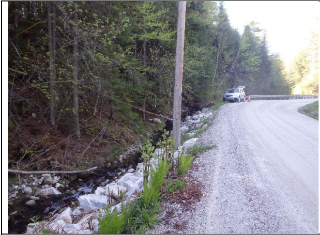
Photograph 37. Roadside stream T-LU-S20 on East Lake Road Ludlow, VT
