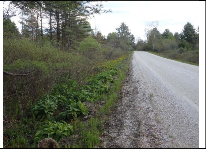
Photograph 38. Pettiner Hill Road, Near Wetland T-LU-W-4, in Ludlow, VT
