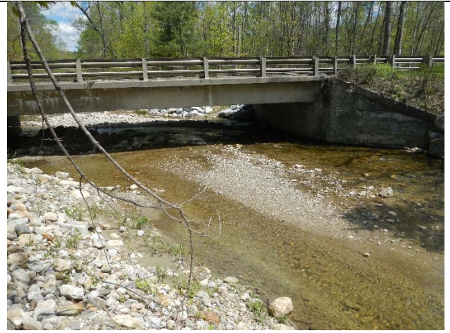
Photograph 26. View of bridge on VT 103 over V-WA-S-4 (Freeman Brook) in Wallingford, VT
