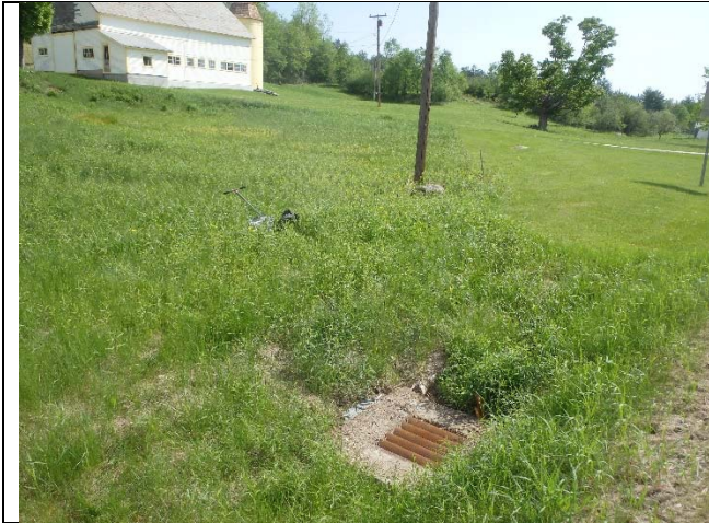
Photograph 31. Residential area along VT 103 in Mount Holly, VT
