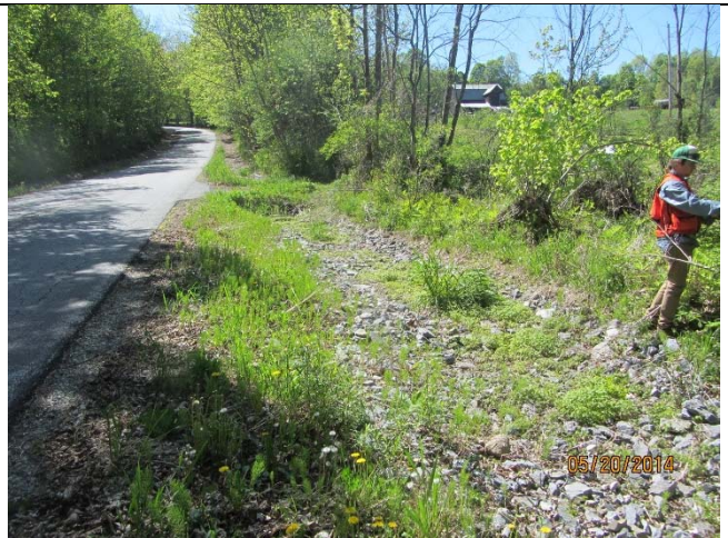
Photograph 8. Hullet Hill Road in Benson, VT
