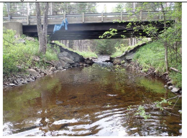
Photograph 30. View of bridge on VT 103 over T-MH-S-28 in Mount Holly, VT (Unnamed Tributary to the Mill River)
