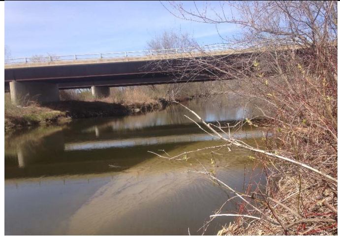
Photograph 18. View of bridge on U.S. 7 associated with T-RU-S-2 (Otter Creek, looking downstream) in Rutland, VT
