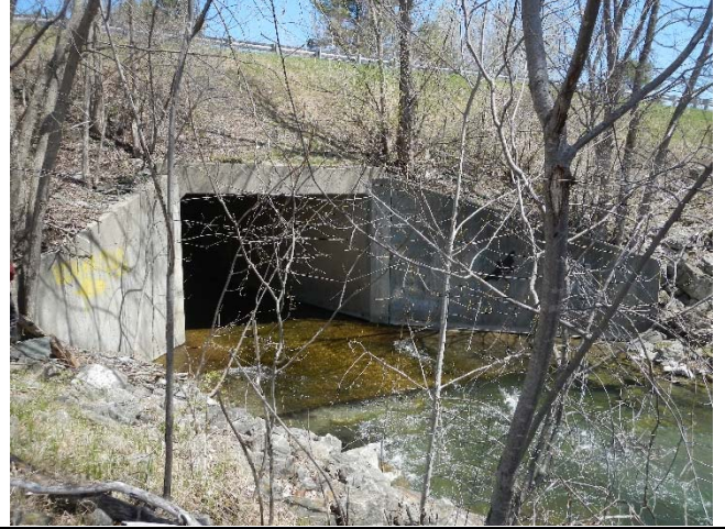
Photograph 16. View of box culvert under U.S. 4 in Castleton, VT
